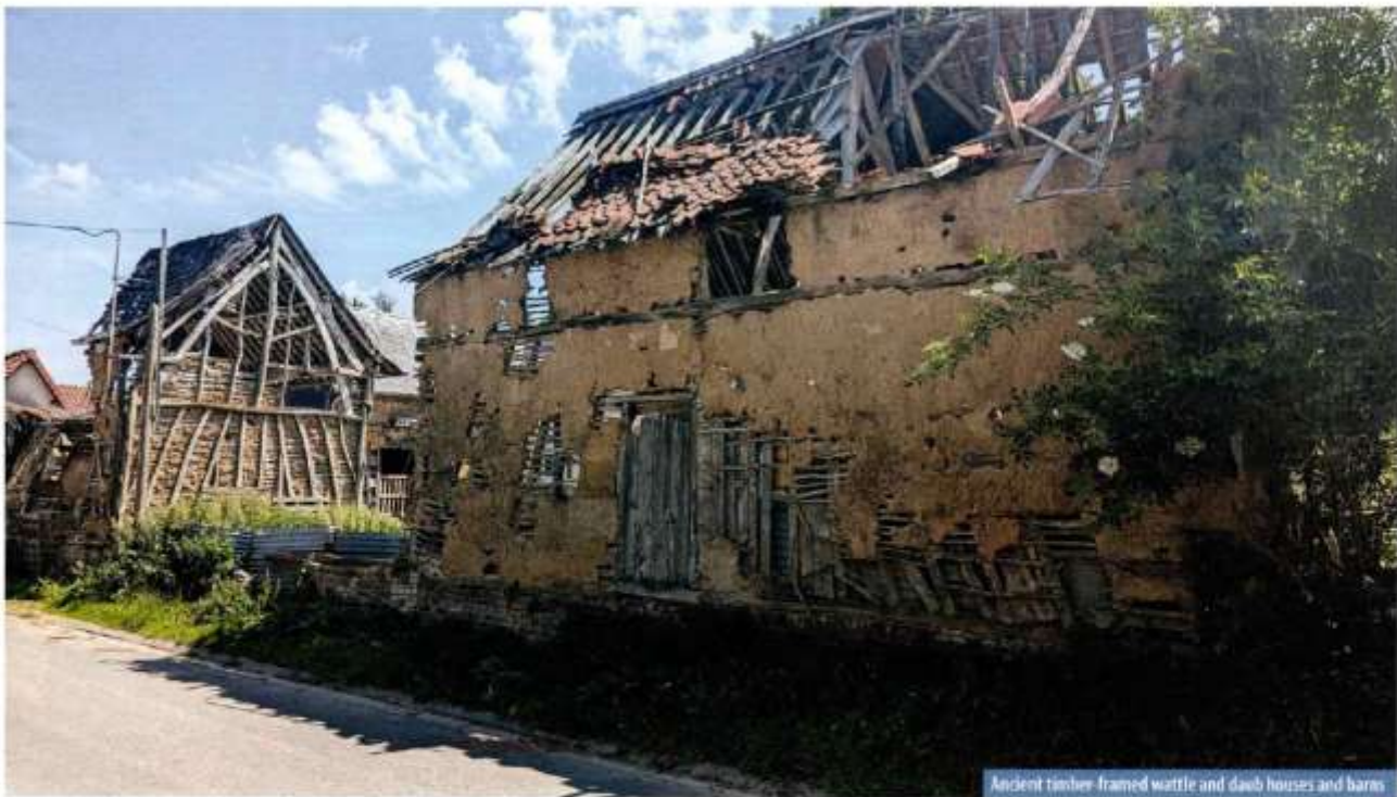
Ancient timber-framed wattle and daub houses and barns
